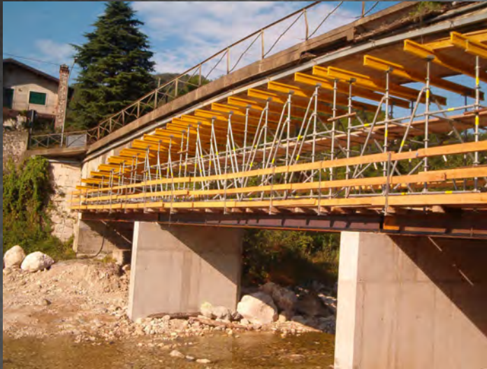
Calvene bridge - Cosfara (IT)
