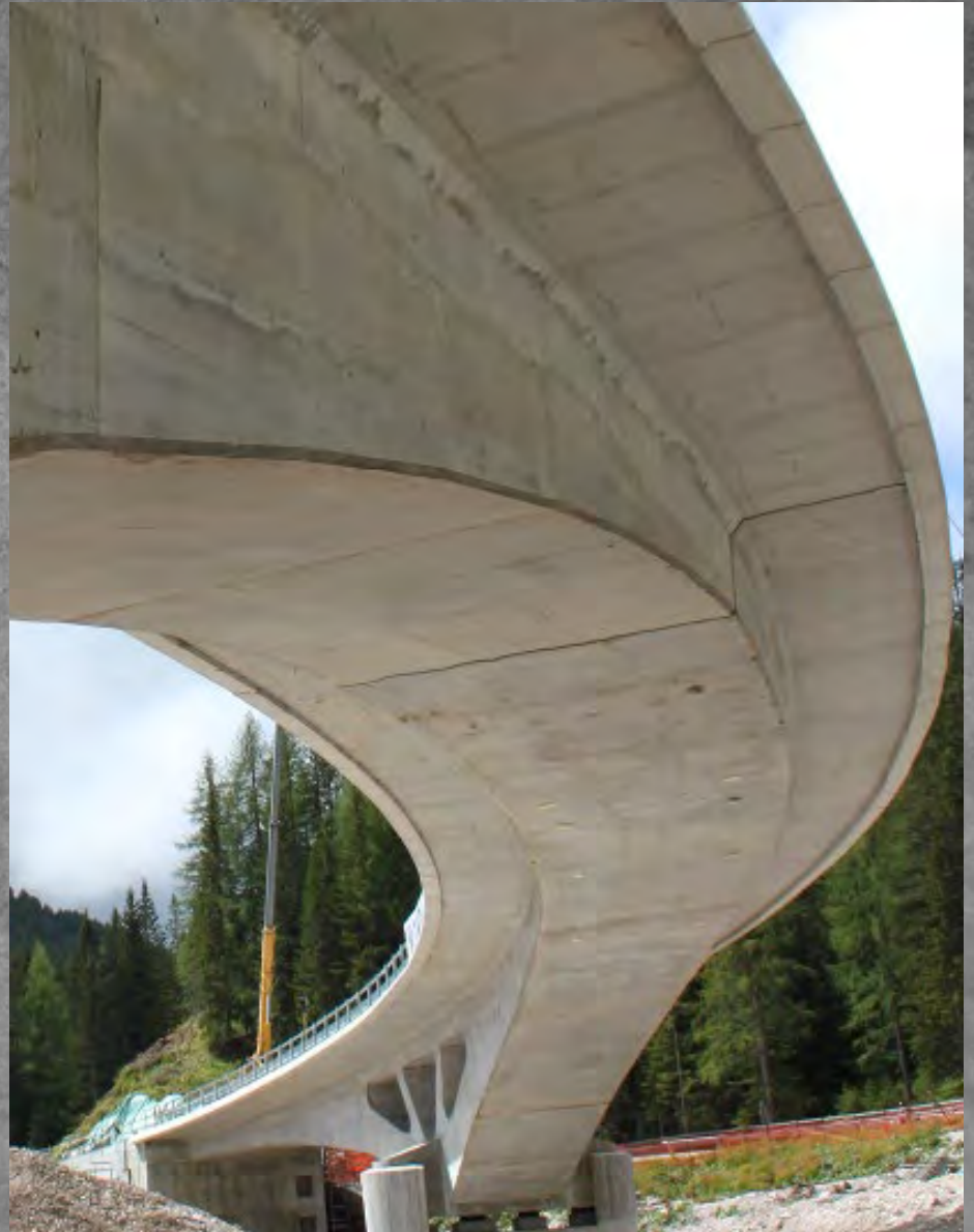
Rudavoi bridge - Cortina (IT)
