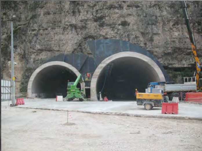
Mezzolombardo tunnels (IT)
